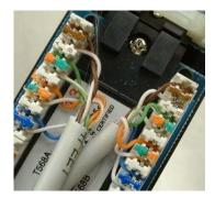
e. The following figure shows a large punch down patch panel with carefully routed cabling.
